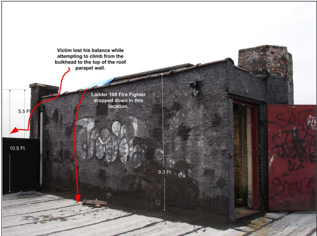
Photo 4. Bulkhead on Roof of Incident Structure. (NIOSH photo)
