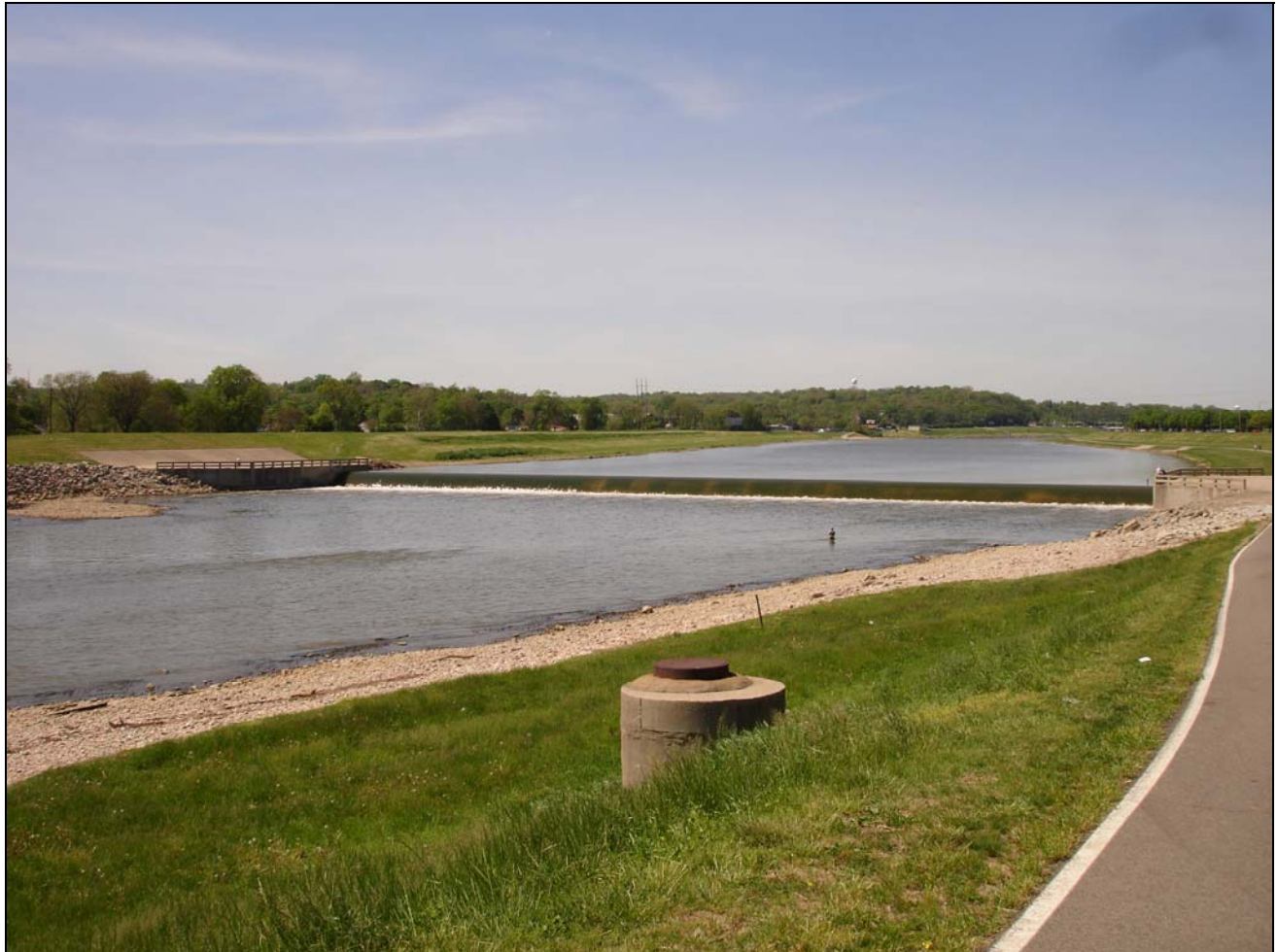
Photo 2. Incident location. (NIOSH photo.)
