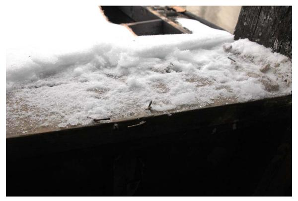
Photo 8. Nails that were exposed at the window sill on the third floor landing.
