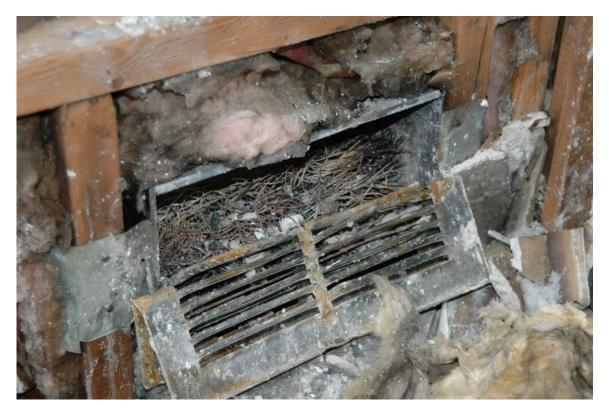
Photo 5. Excelsior that was stuffed into duct work vents.
