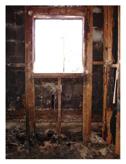
Photo 4. Window sill on third floor landing looking towards the rear or C-side of the structure. Sill is 41-inches above floor level
