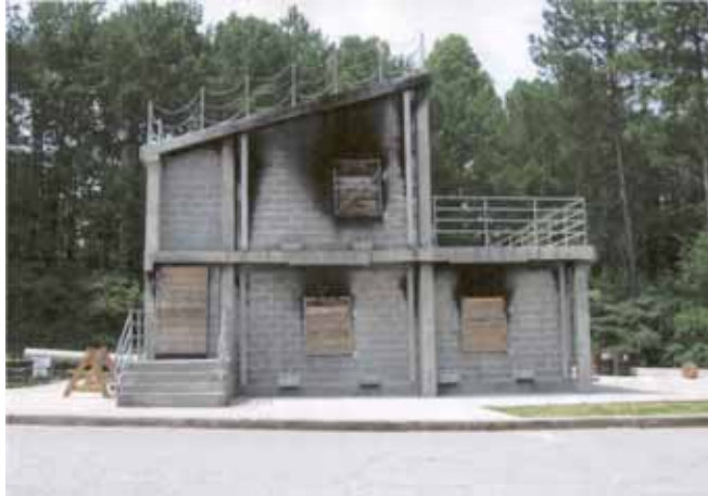
Photograph 1. Fire Training Structure
