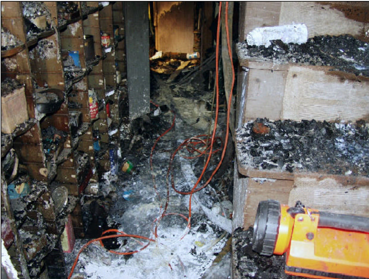
Photo 1. Narrow hallway at bottom of basement stairs.
