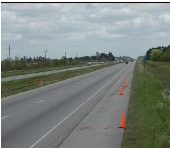
Interstate highway eastbound lanes
