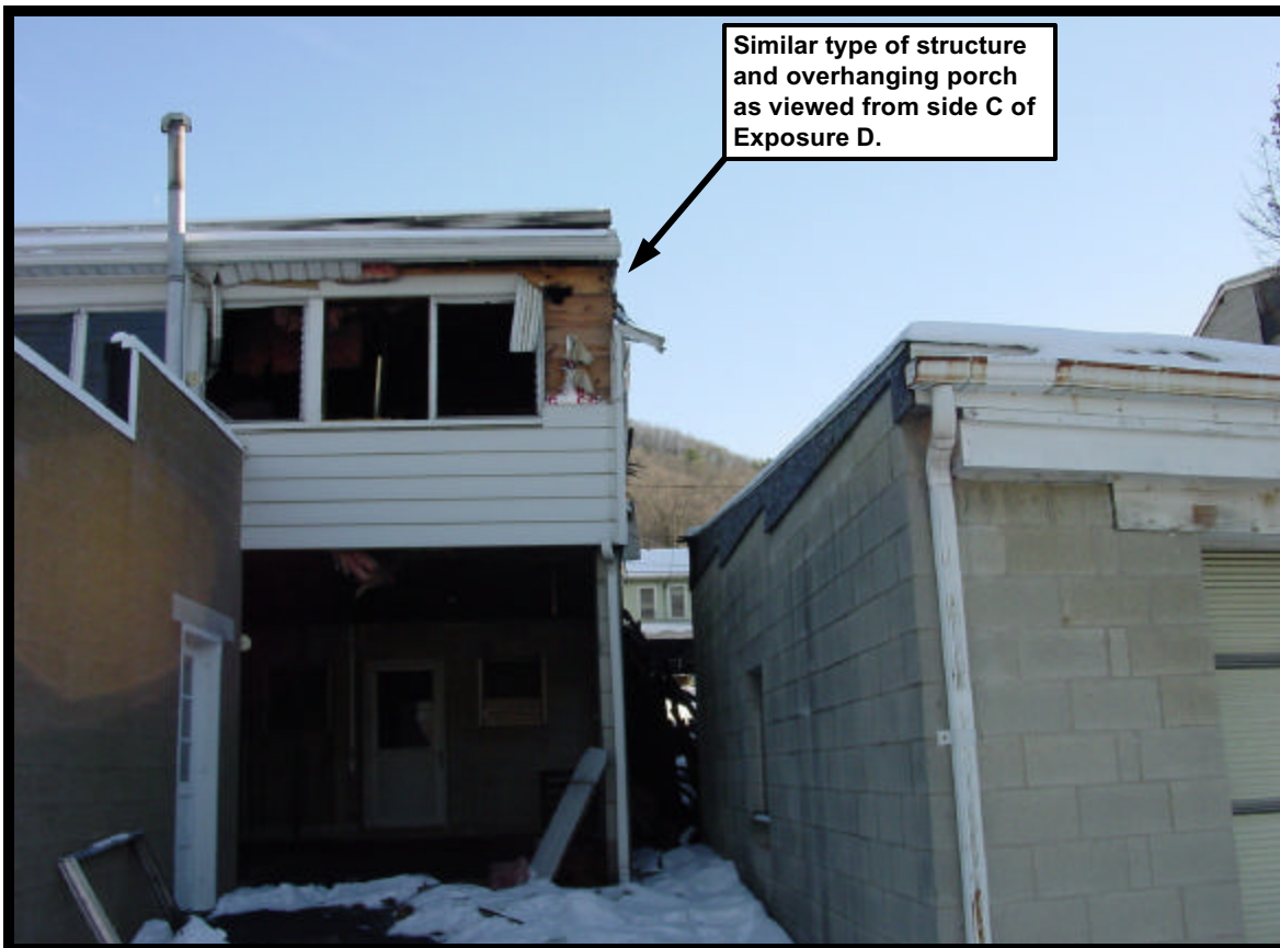
Photo 1. Rear Porch, Exposure D
