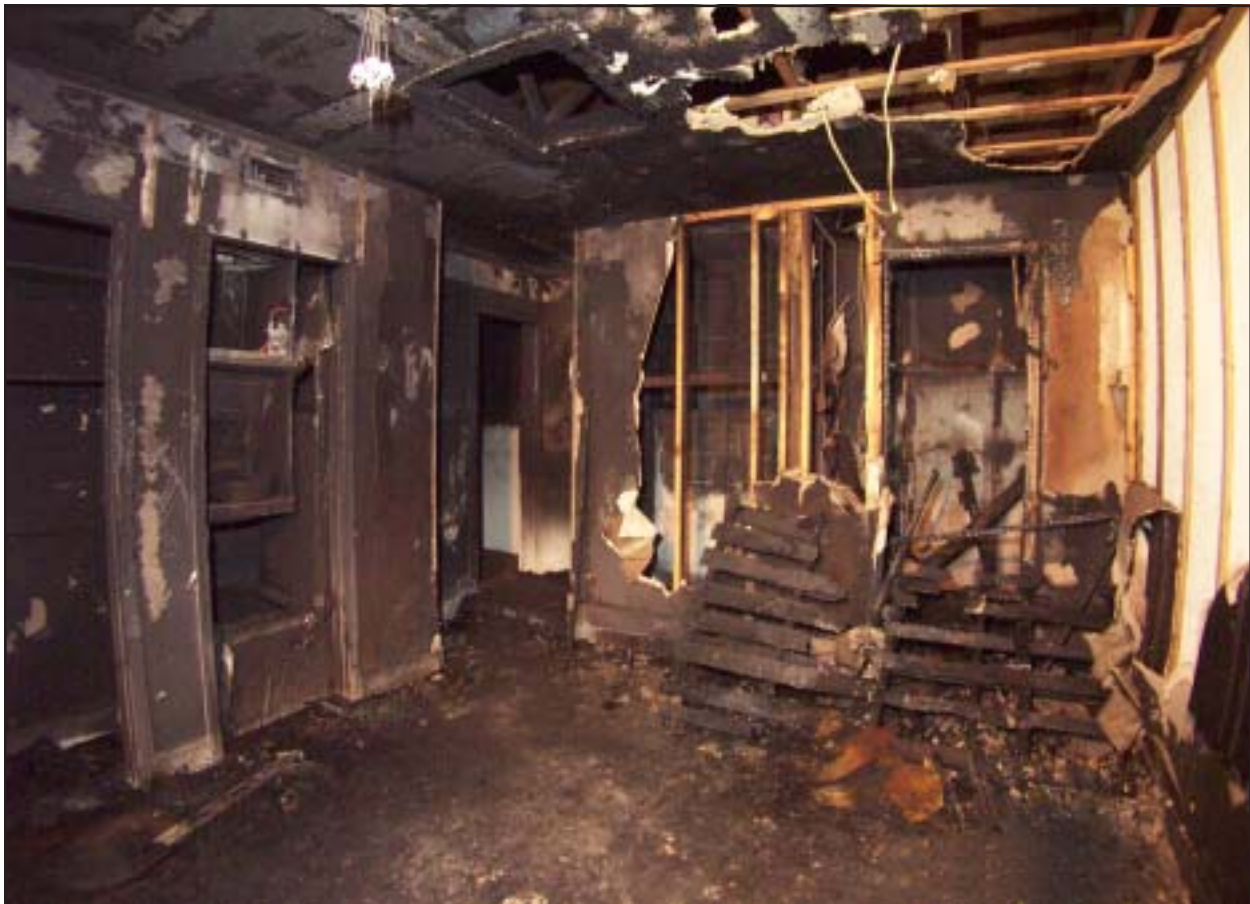
Photo 2. Burn room in the structure
