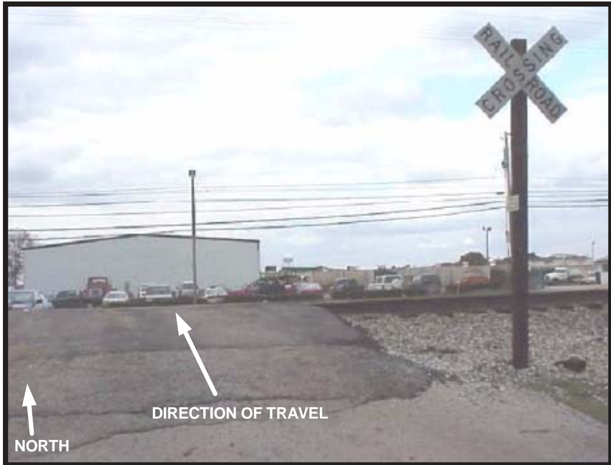
Photo. Northbound View of Incident.
