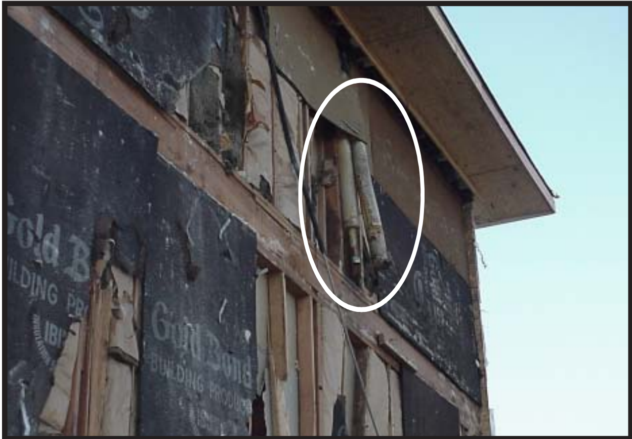
Photo 3. Water Pipes; Originally Covered by a Section of Brick Veneer
