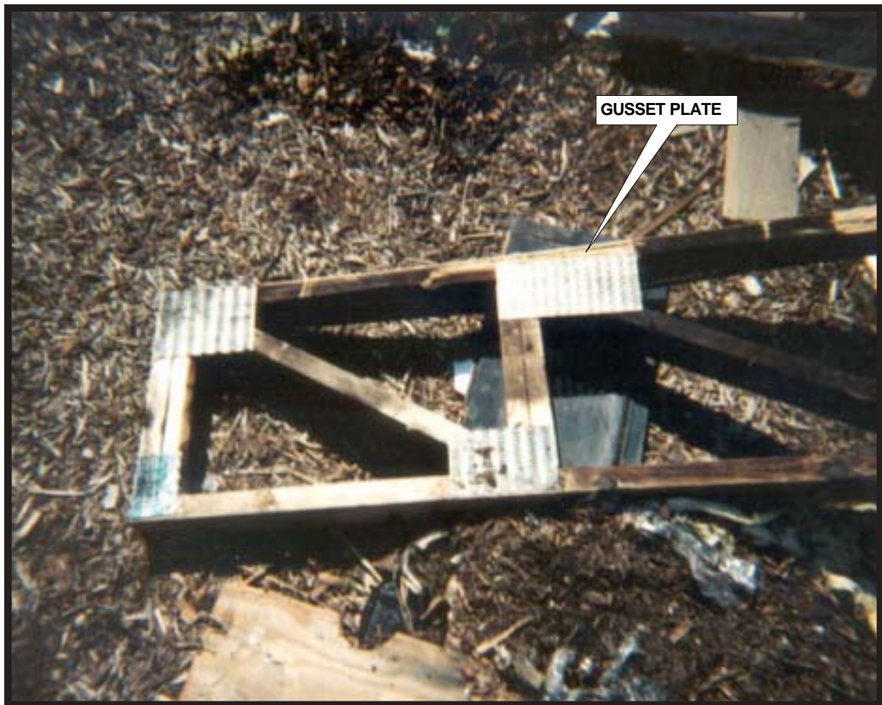
Photo 2. Lightweight wooden parallel-chord truss
