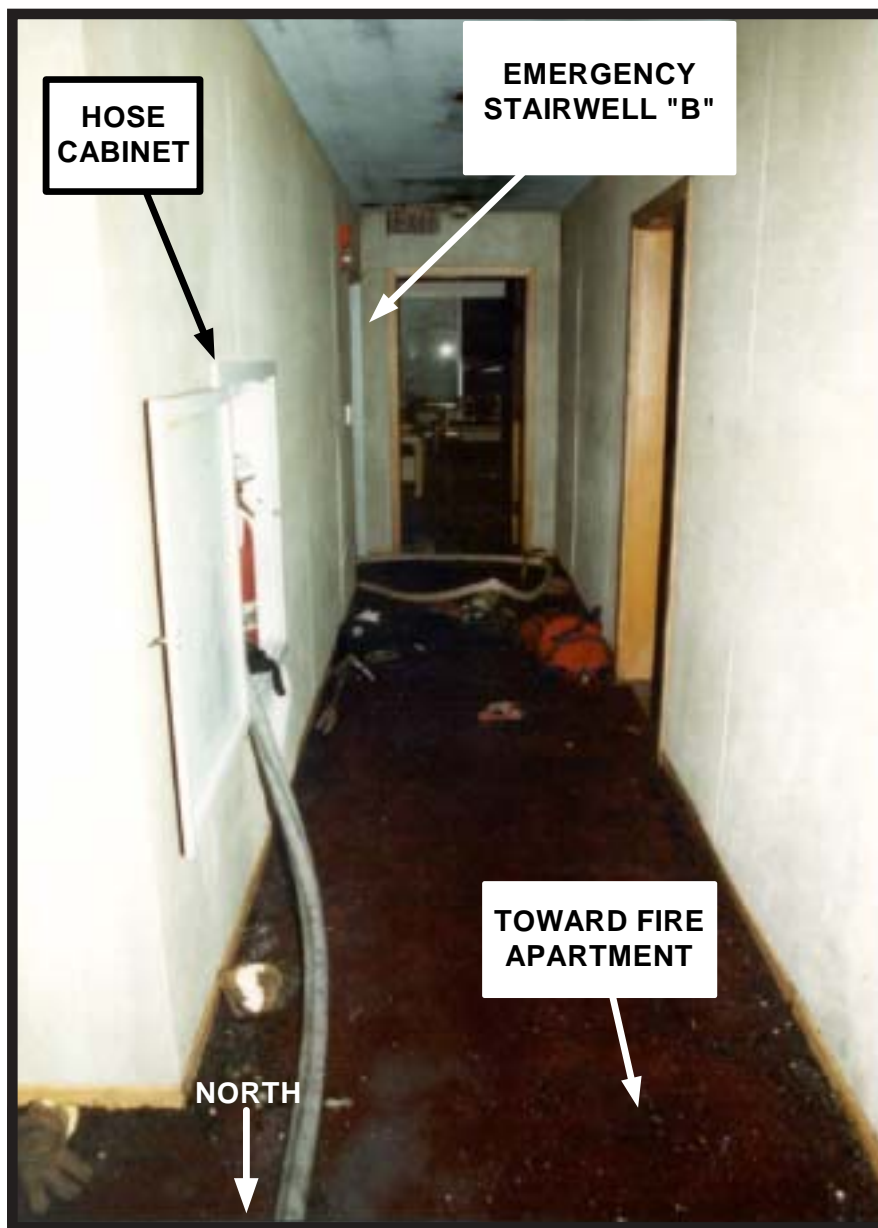
Photo 3. View of Hallway Leading Toward Emergency Stairwell “B”
