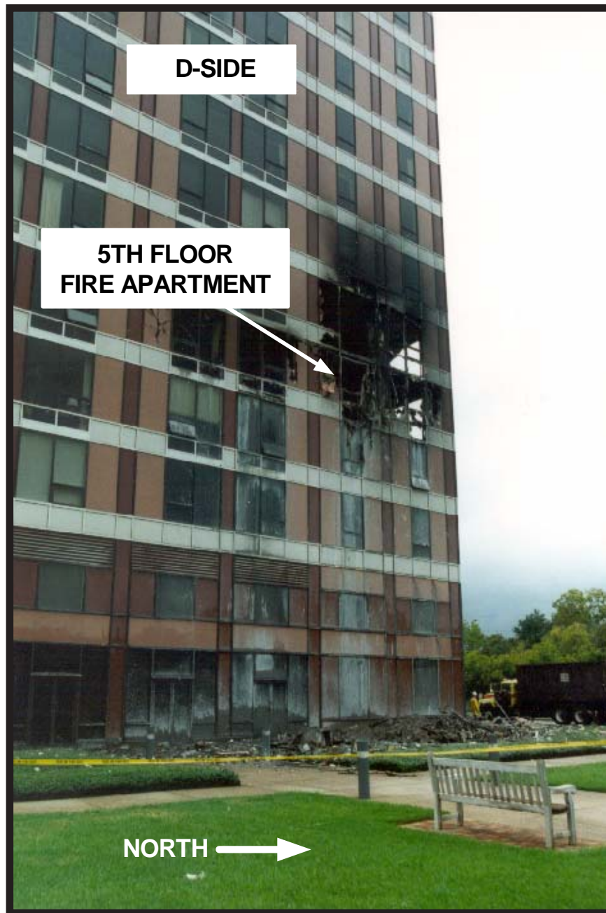
Photo 2. View of D-Side of Building
