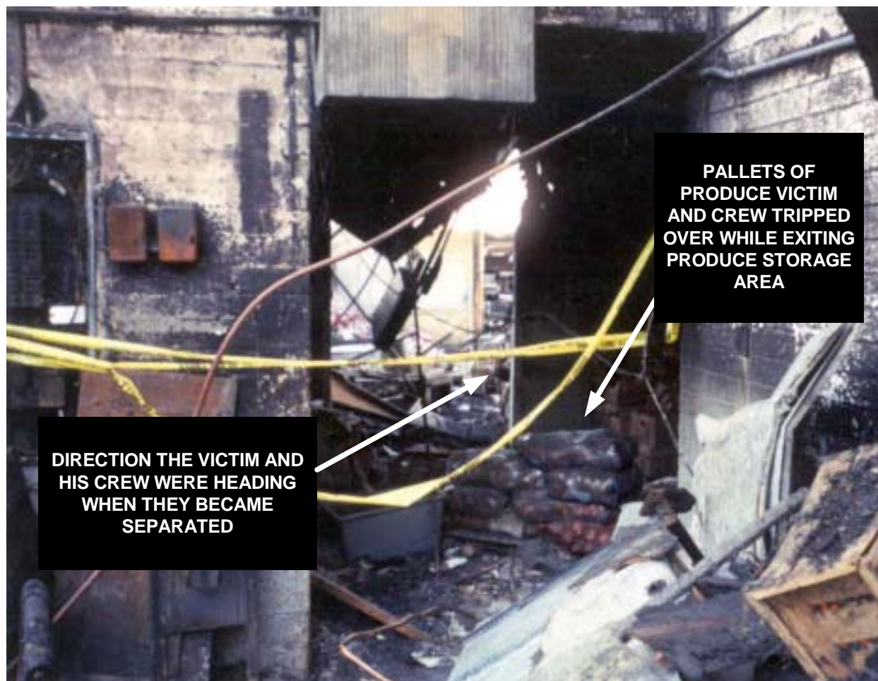
Photo 3. View of Produce Storage Area
