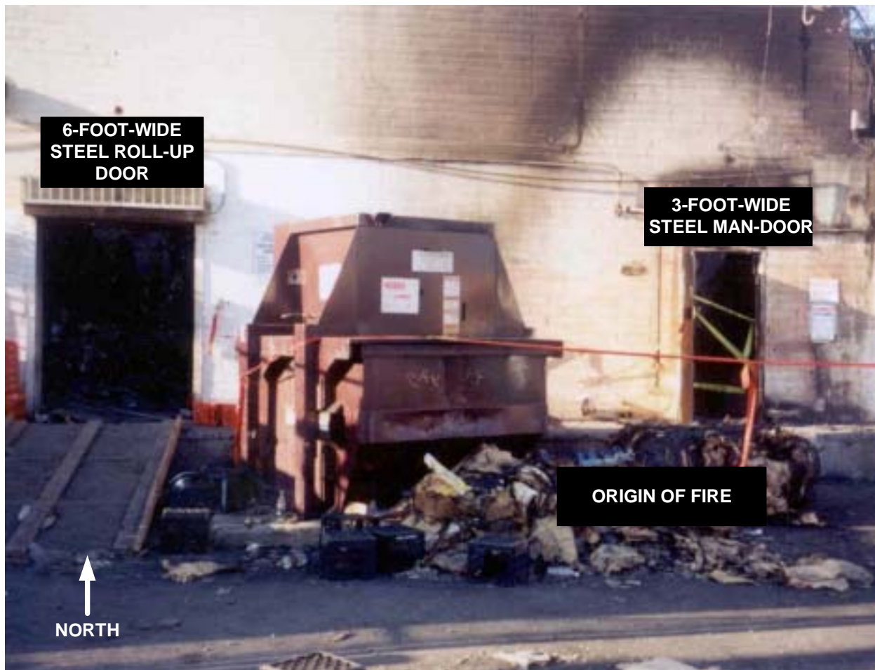
Photo 1. South Entrances of Supermarket
