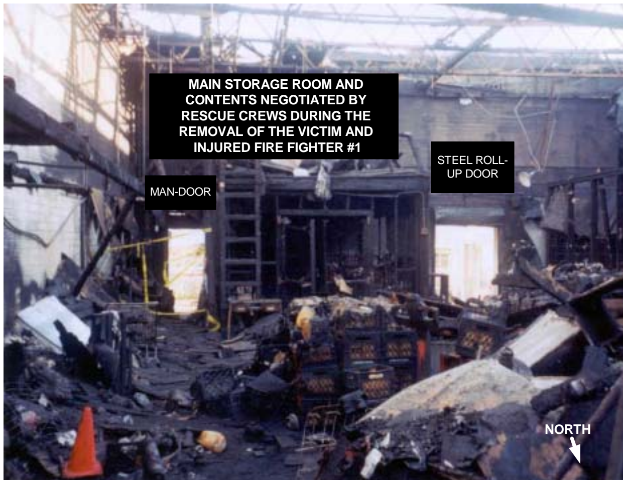
Photo 2. Main Storage Room
