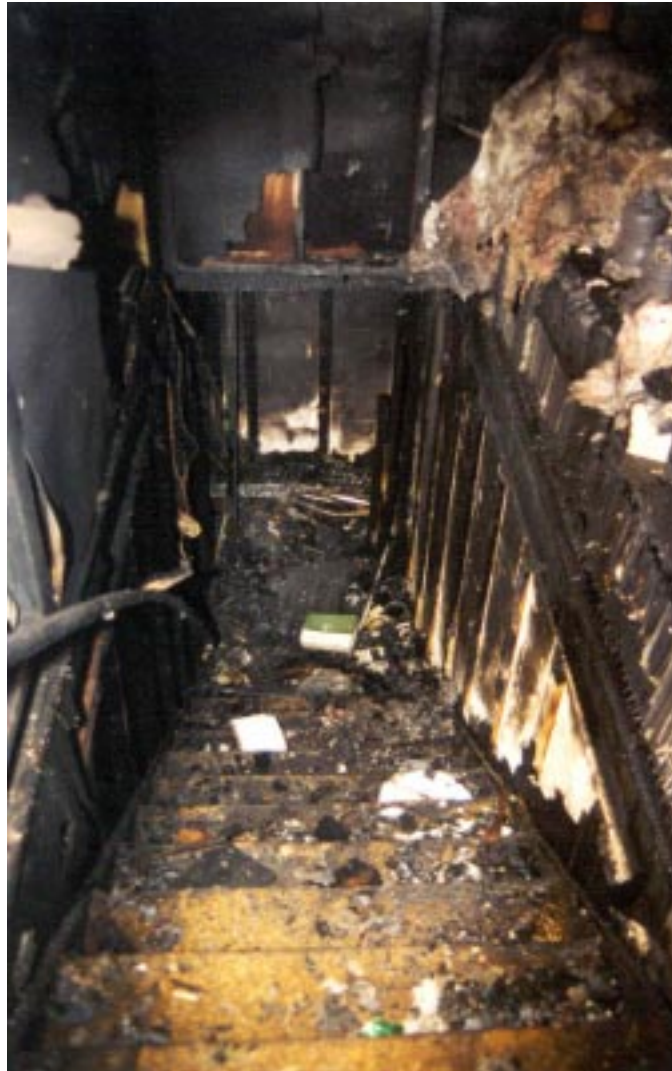
Photo 7. Stairway Connecting Addition to Basement
