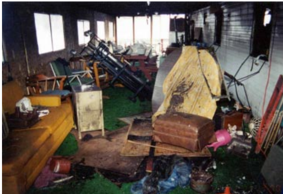
Photo 2. Enclosed Porch Attached to Mobile Home
