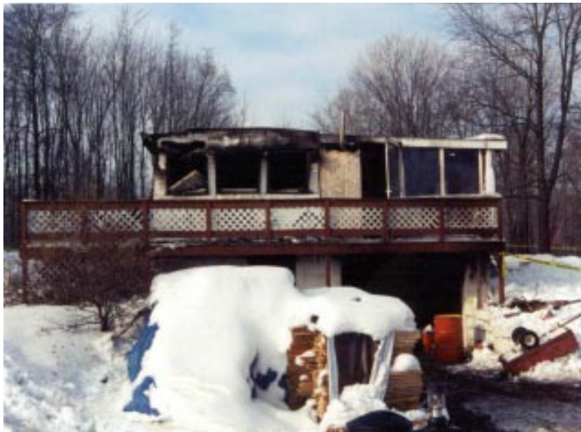
Photo 5. Entrance to Garage and Basement Area (Side 2)
