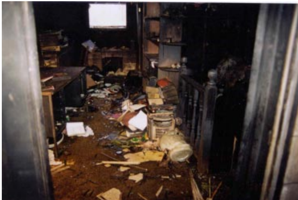
Photo 3. Addition to Mobile Home (12 ft x 12 ft)
