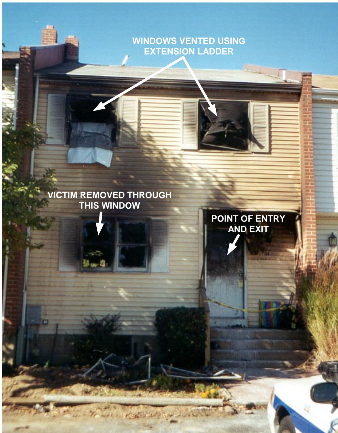
Photo 1. View of Side 1
