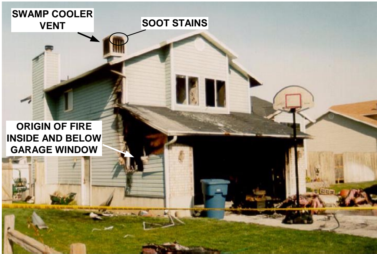
Photo 2. Street View of Incident Scene
