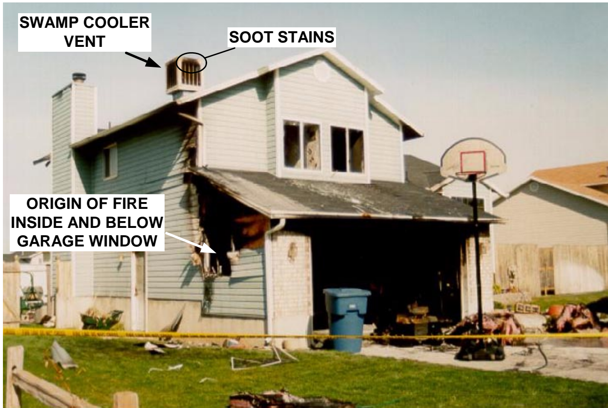
Photo 2. Street View of Incident Scene
