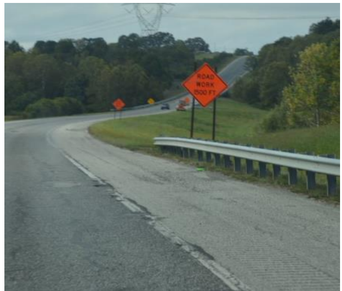
Photo 4. Photo showing second work zone sign present as you approach the scene of the incident traveling east. Sign reads, "ROAD WORK 1500 FT."
