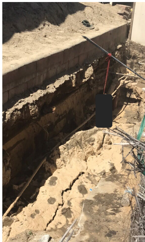
Exhibit 3. The trench after the water was removed. Photo by CA/FACE program.
