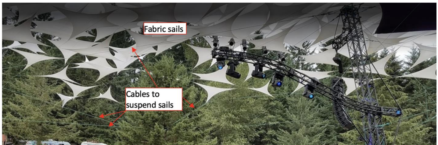
Image 1. Image of a fabric sails installation at the music festival venue. Note the cables attached to the sails are secured to trees in the background.
