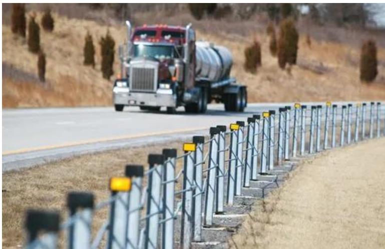
Photo 7. Photo depicting standard installation of median cable barriers on an interstate highway 11 .
