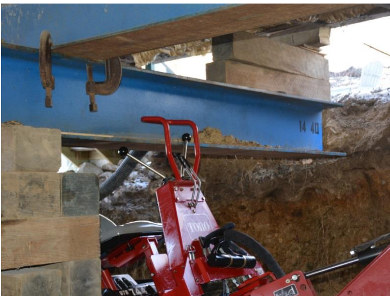
Figure 7 – The excavator's left control lever against the overhead beam
