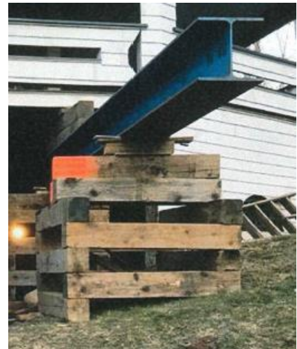
Figure 2- Steel support beam and cribbing
