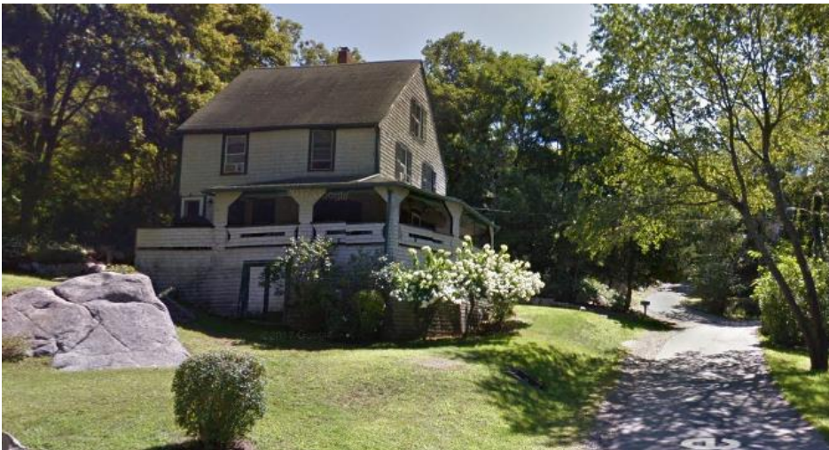
Figure 1 - View of home, facing uphill, before work began
