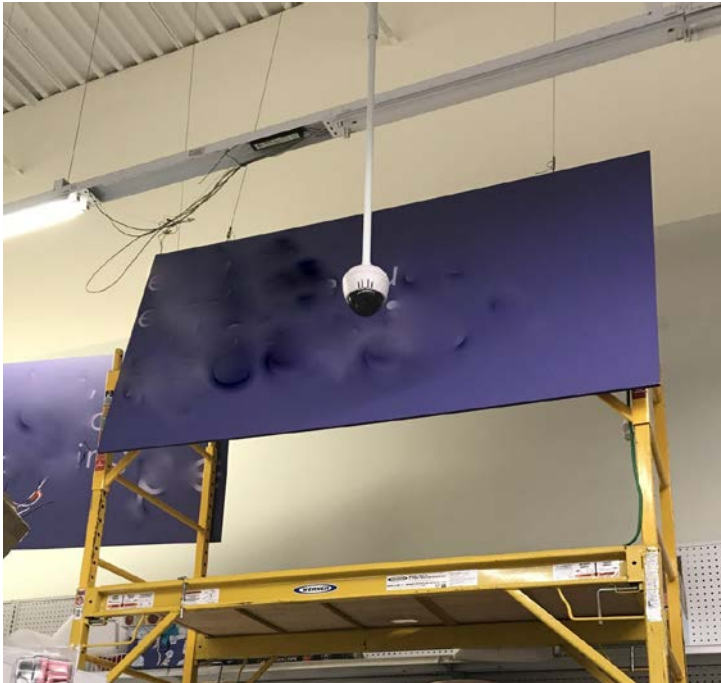
Image 6. Light fixtures and signage suspended from the roof by metal braided wire. Scaffold location recreates where decedent was working at the time of the incident. Writing on signs obscured for report.
