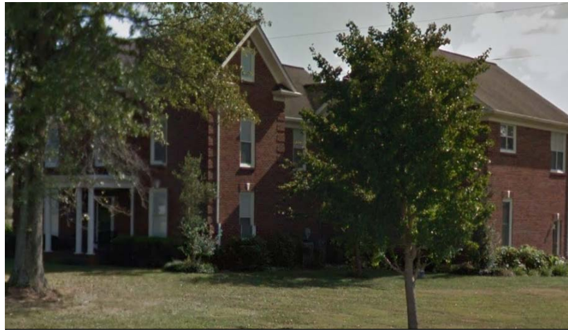
Image 1. Residence the victim was working on at the time of the incident. Photo property of KY FACE.
