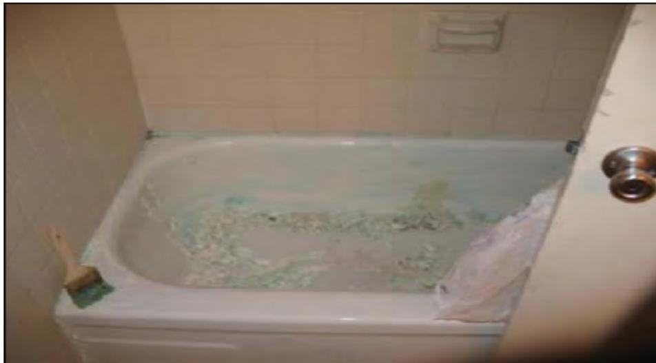
**Exhibit 1.** Photo of a similar bathtub being stripped of paint using a chemical paint remover (not the bathtub in this incident). *Photo courtesy of Michigan Fatality Assessment and Control Evaluation program.*
