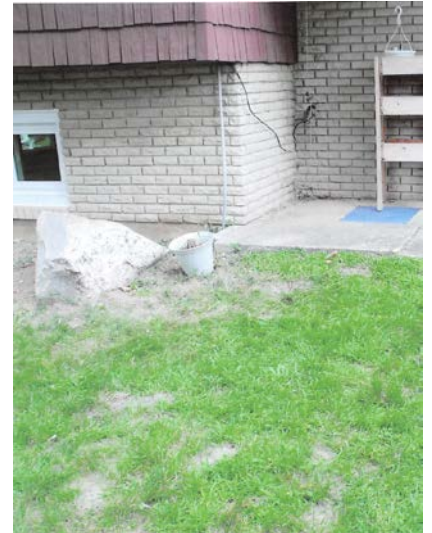
Photo 3. Area to which to decedent fell
