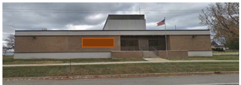
Photo 1. Front of water treatment plant undergoing renovation.
