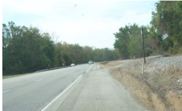
Figure 3. Shoulder where the incident occurred.
