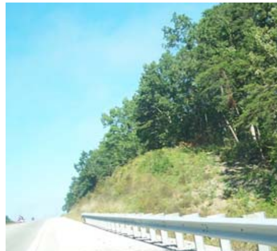
Figure 1. Highway shoulder; approximate location of the collision.
