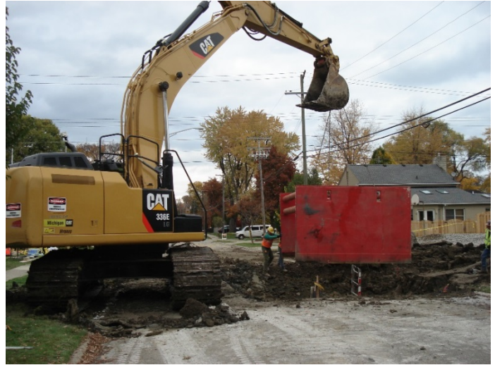
Figure 2. Placement of trench box after road removal
