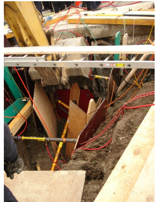
Figure 1. Recovery operations trench wall support
