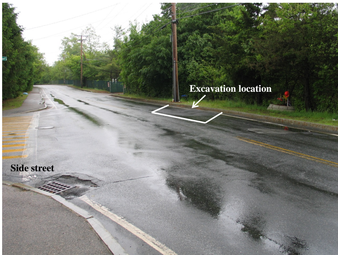
Figure 2 – Roadway view of the T-shaped intersection with excavation location outlined
