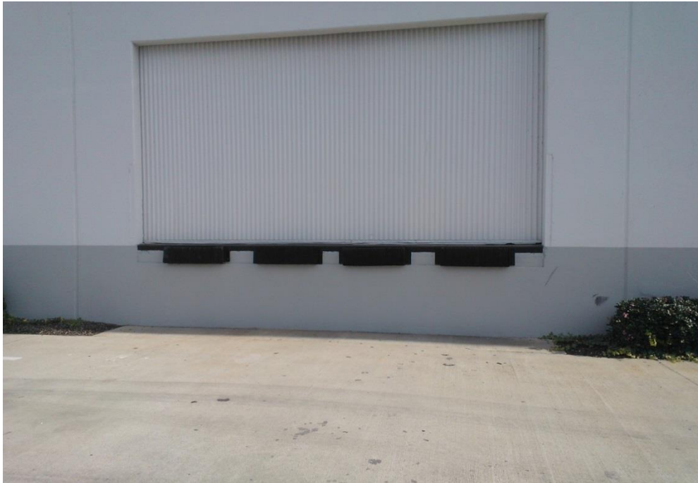
Exhibit 1. A truck loading dock identical to the one involved in the incident. Trucks back up to the dock in order to load and unload product.
