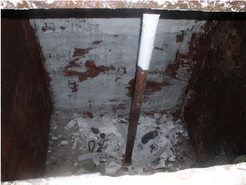
Exhibit 4. The interior of the paint tank.
