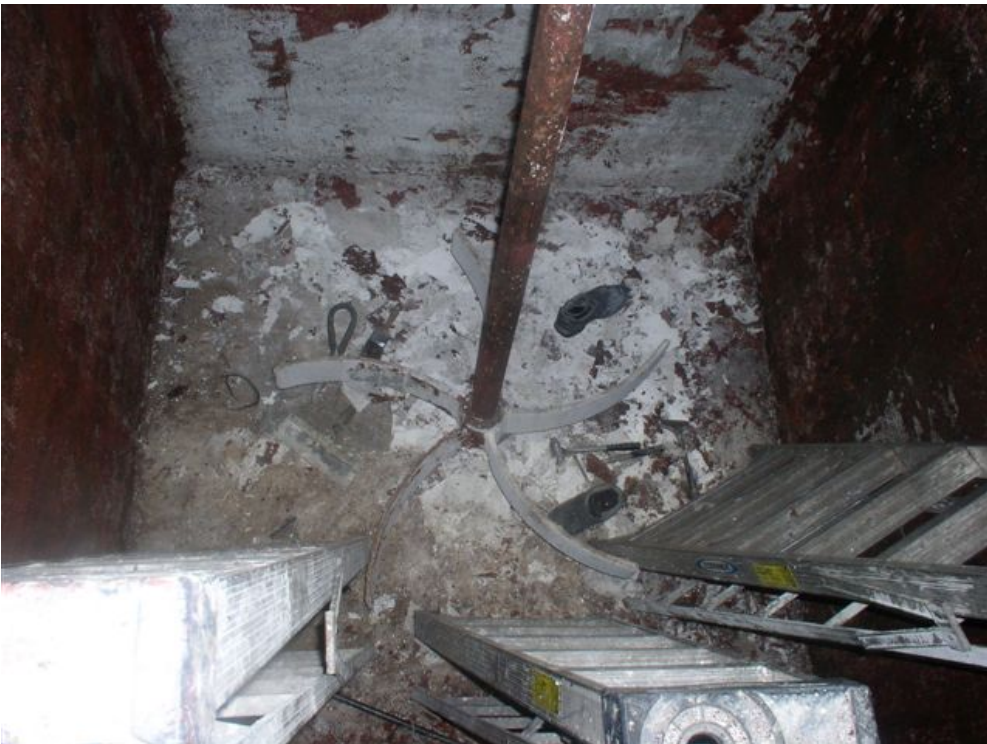
Exhibit 5. The ladders used to enter the tank.
