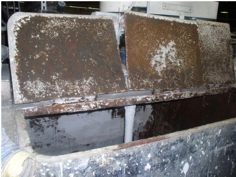
Exhibit 3. The paint tank opening.
