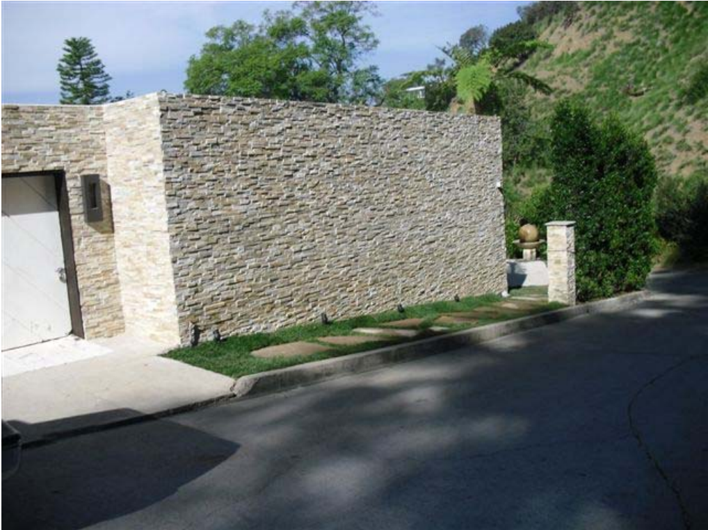
Exhibit 1. The stone and stucco work at the incident site.
