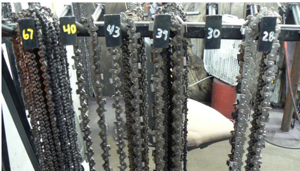
Photo 15: Numbered rack in maintenance shop. Chains on rack have been inspected and are waiting to be put into orange bins with motor oil. Rack is locked to ensure that equipment operators cannot take chains from rack.
