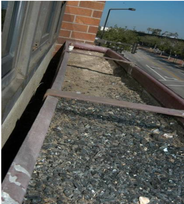
Exhibit 7. The separation between the building and another planter box.
