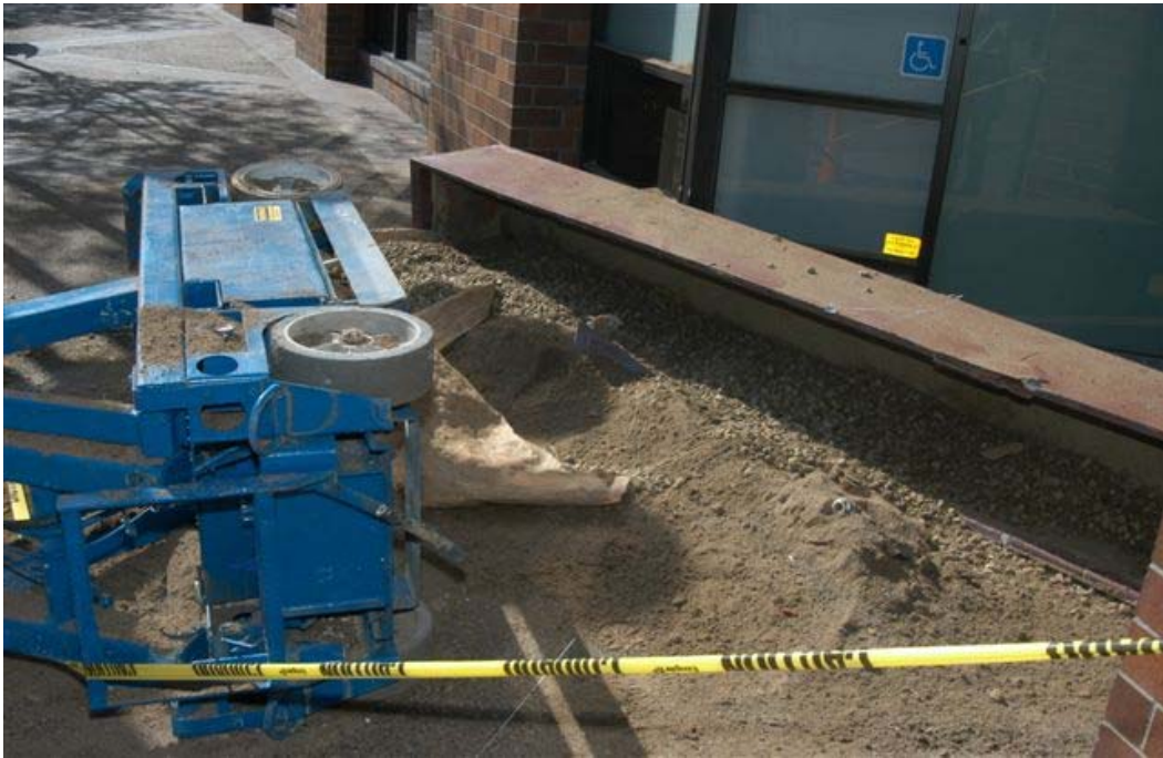
Exhibit 6. The dirt and gravel that was in the planter box when it fell off the ledge.
