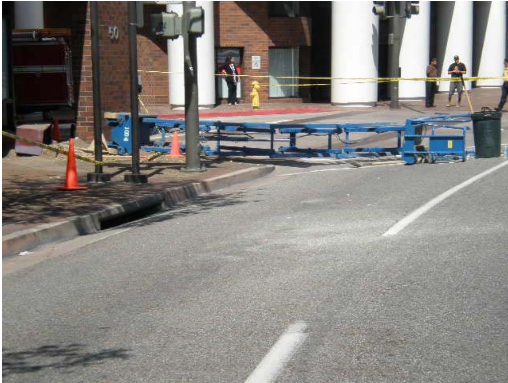
Exhibit 1. The toppled scissor lift.
