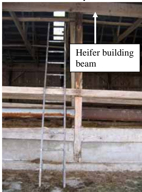
Figure 4. Ladder placed under (not supported) by the building beam and against fence railing
