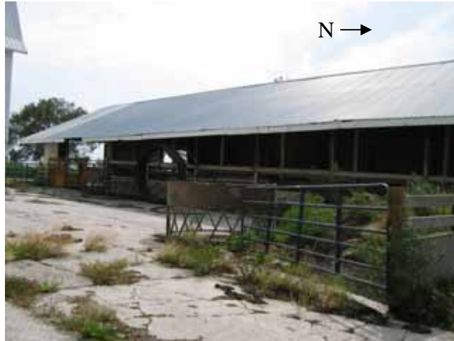
Figure 1. View of incident scene
