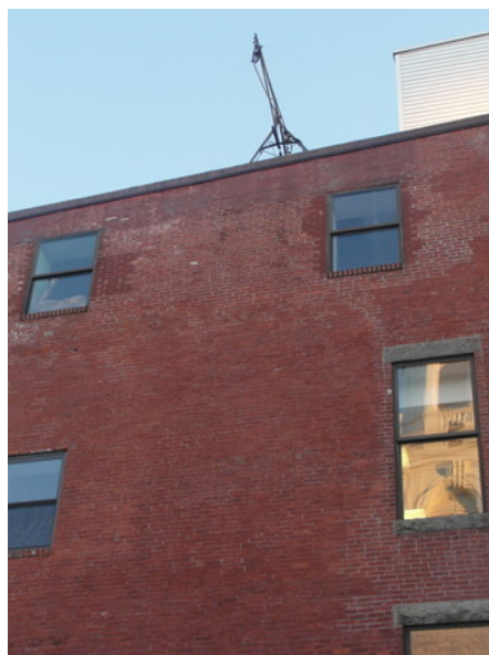
Figure 2 – Building with the pulley system being used during the incident
