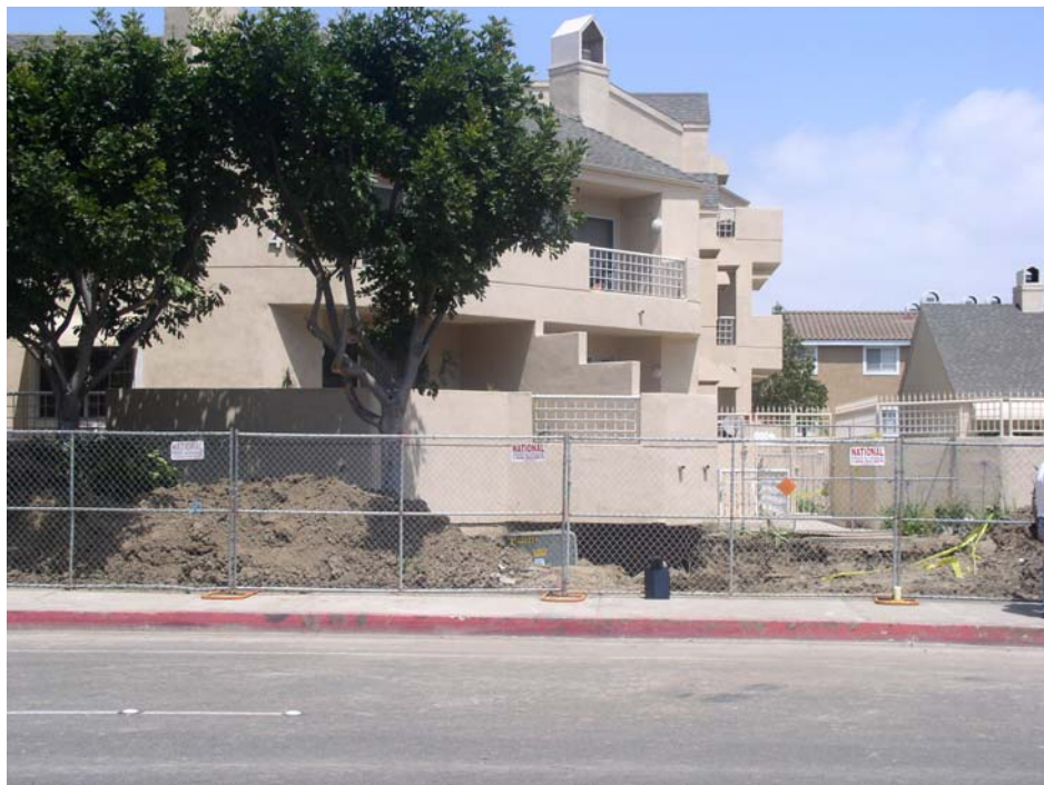
Exhibit #1. The apartment complex where the incident occurred.
