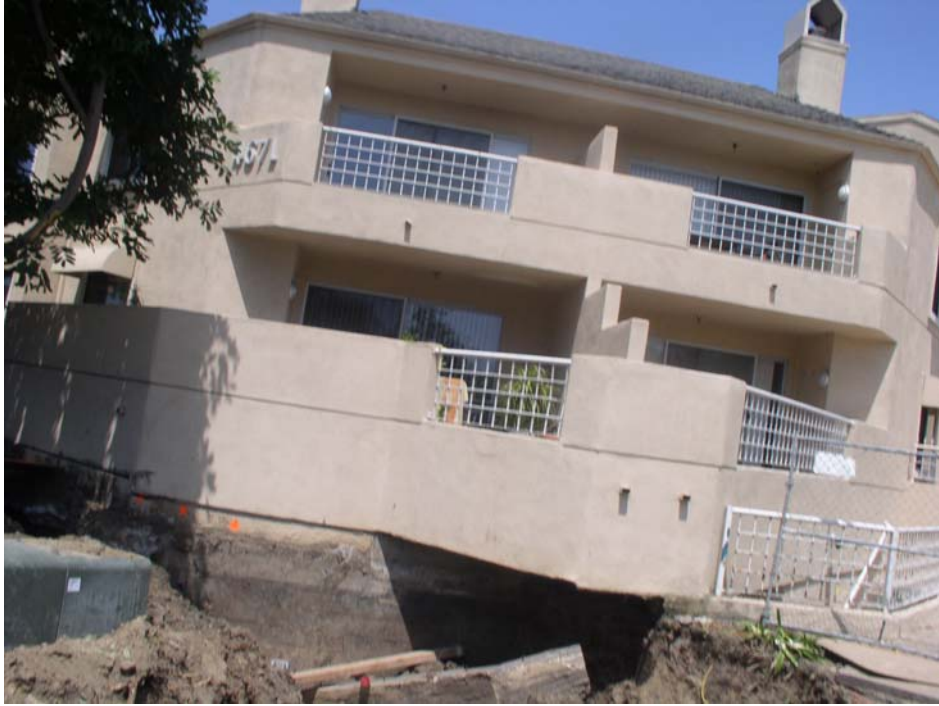
Exhibit #2. The two apartment patios affected by the excavation.
