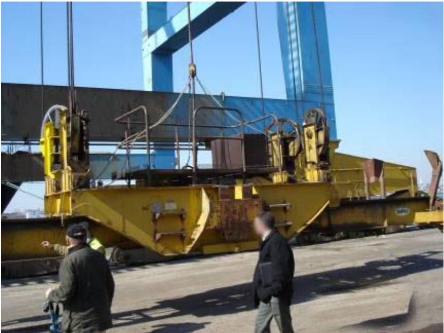
Figure 2 - The spreader involved in the incident lowered to the approximate height for lubrication of the guide rails.
