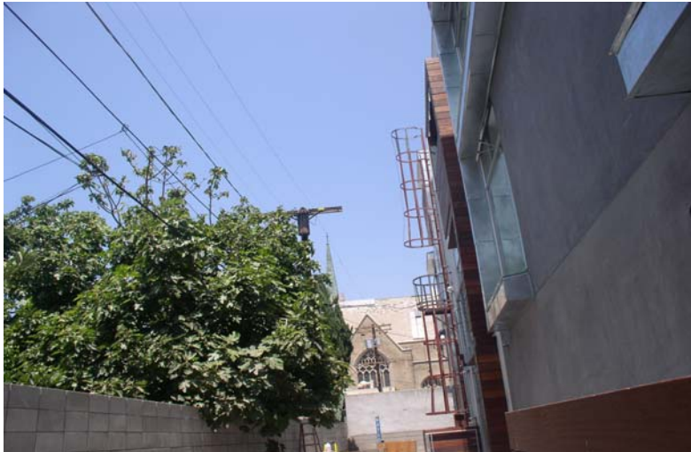
Exhibit 1. The high voltage lines in relation to the building under construction.
