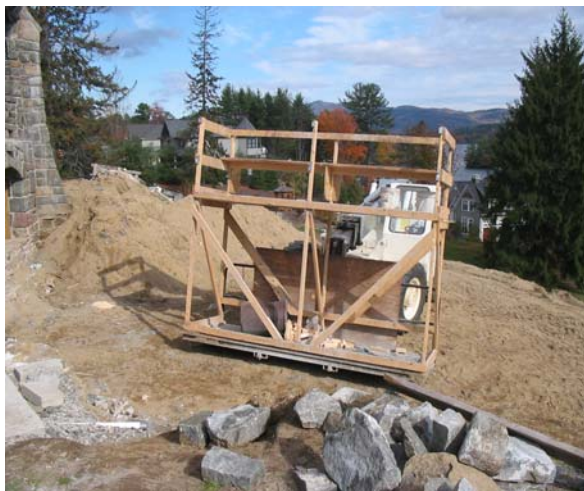
Photo 4 Two-tier Platform (courtesy of OSHA)
