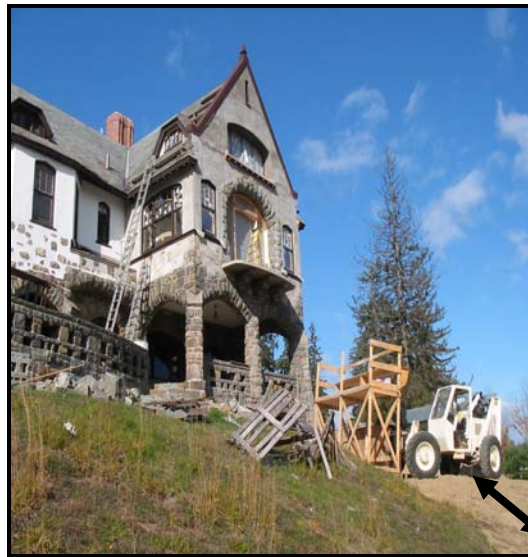
Photo 2 Sloped terrain (courtesy of OSHA)
