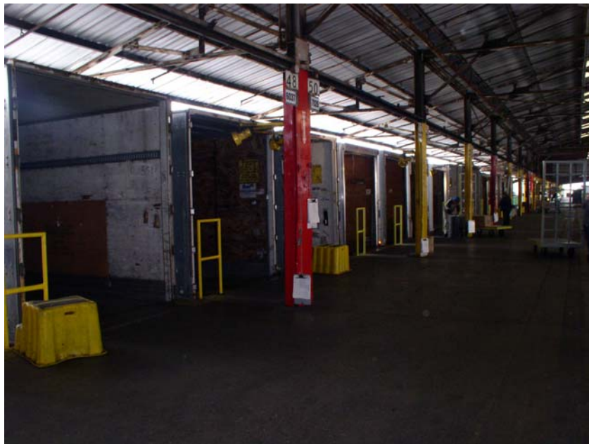
Exhibit 5. The receiving dock with trailers waiting to be loaded.
