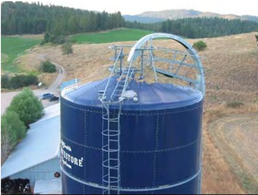
Photograph 1. A view of the top of the silo with ladder cage and chute extended after filling.
