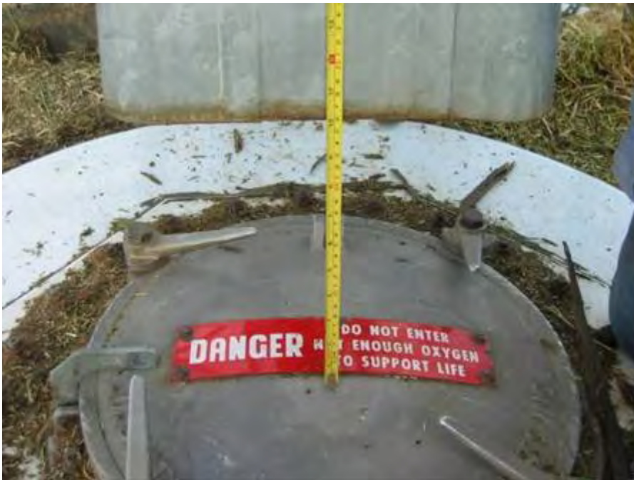
Photograph 2. The silo access hatch on the top of the silo.
