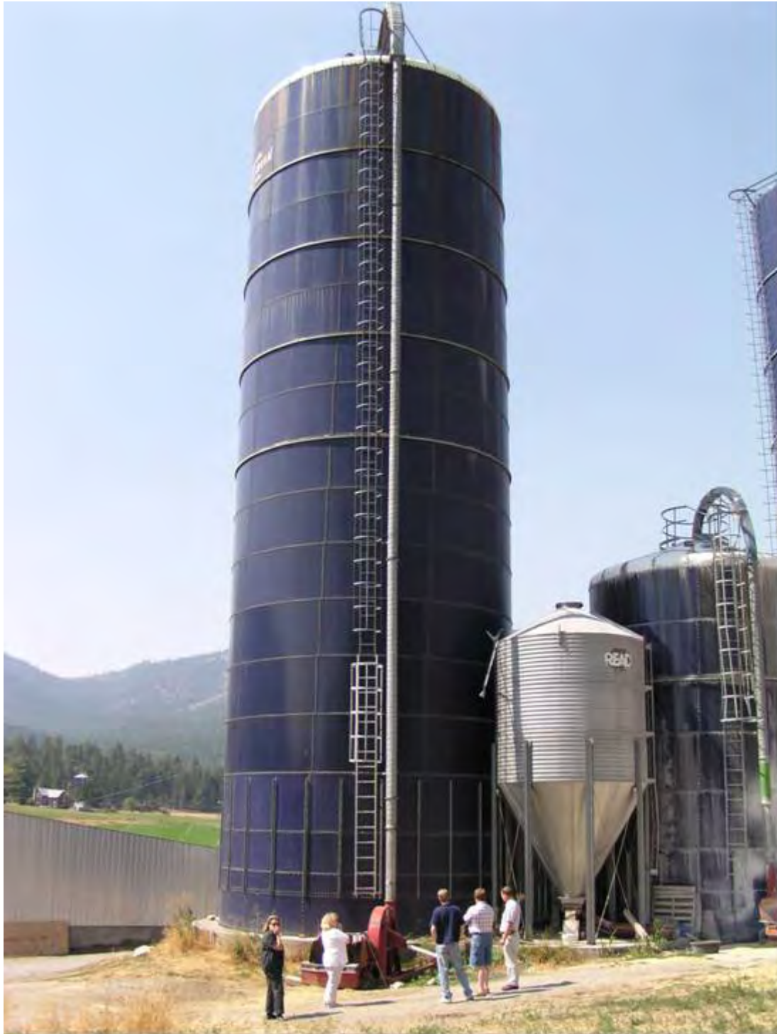
Photograph 3. A view of the silo from ground-level.
