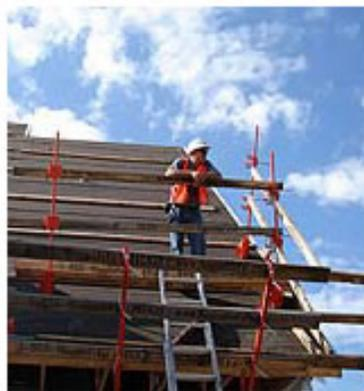
This photo taken by Tom Bobick tied for third place in domestic programs. His photo demonstrates workplace safety. The worker is on a 45° steep-slope roof, notes Bobick. "What is normally a risky workplace has been turned into a safe work environment through the use of the NIOSH-designed adjustable roof bracket-safety rail system..."
