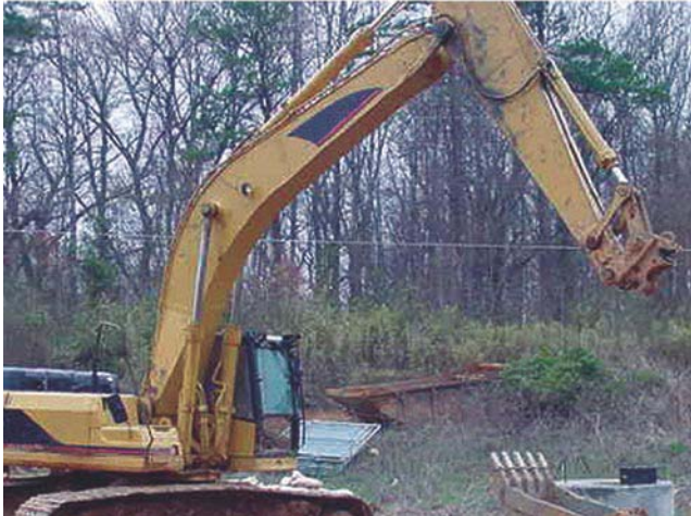
Figure 1. Quick-disconnect excavator bucket that detached from the excavator stick.
