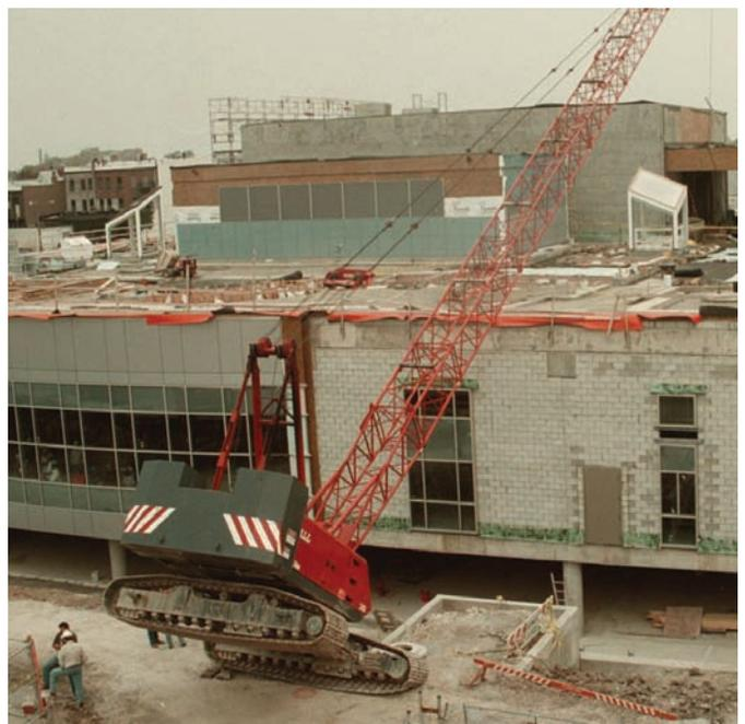
Crane tip-over at library expansion project. (Photo courtesy of The Blade/Toledo Ohio)
