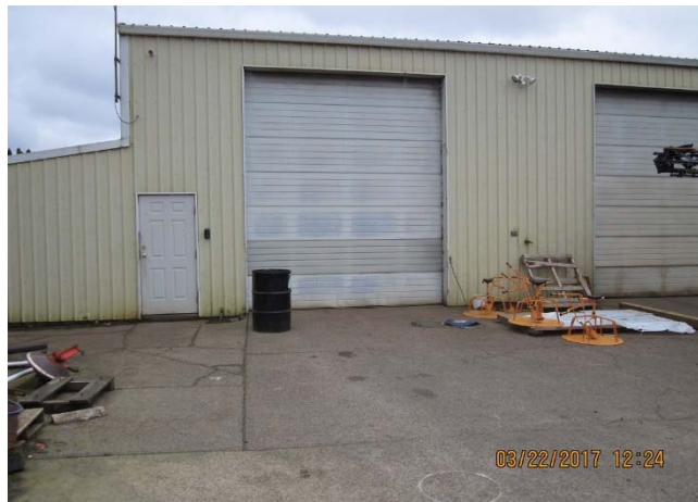
Photo 1. Shop exterior; bay door reportedly had been partway open at time of incident, presumably for ventilation ( Photo courtesy of OR-OSHA ).
