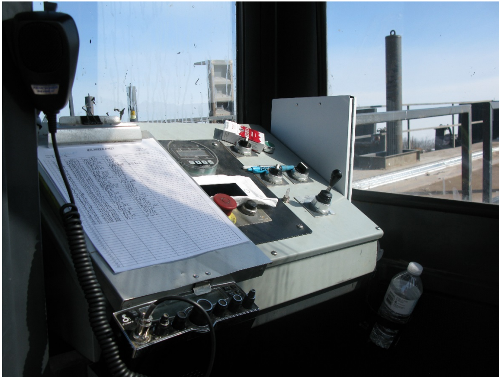
Photo 3. Tipper control panel and a CB radio inside the operator's cab.
