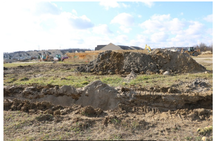
Figure 1. Placement of spoils
