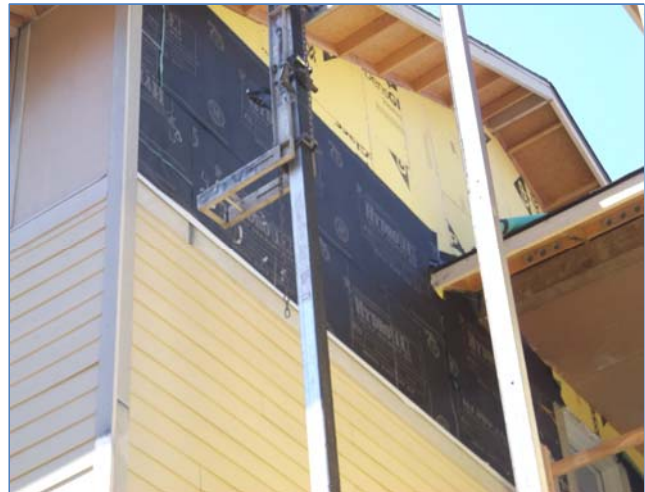
Figure 4. Peak section of breezeway wall.
